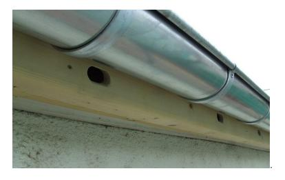
On the left; a simple timber box, with internal partitions, that has been fitted under and behind the gutter to form a continuous array of Swift nest places. The entrance holes are sized to resist access by Starlings.
