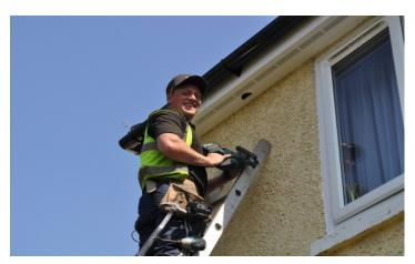
A specially trained workman cuts the right size hole in the right place to let Swifts back into these eaves, where they have been nesting already for many years, after the fitting of new soffits and gutters.
