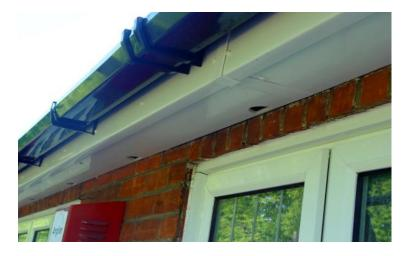
On the left; plastic soffits that have been fitted with internal partitions and drilled with Starling-proof entrance holes for the Swifts to gain access and make their nests inside. These soffits are isolated totally from the roof interior.
