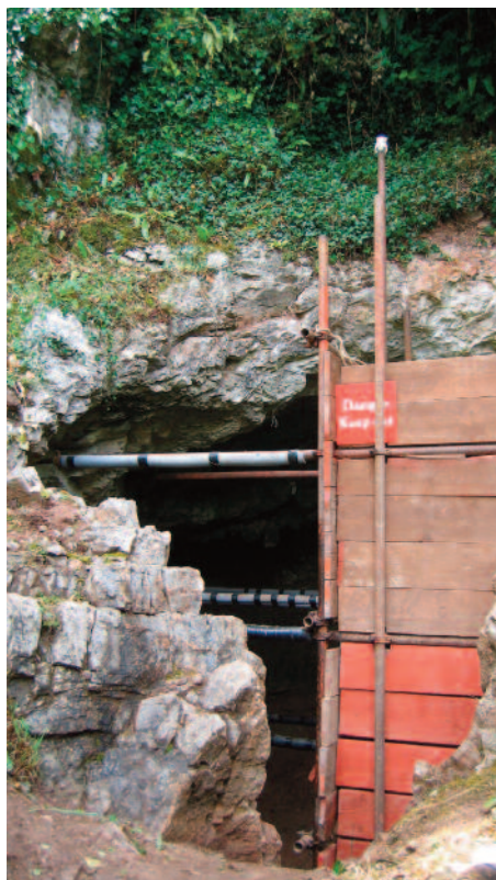
Below, scaffolding and shoring protect the undug reserve
