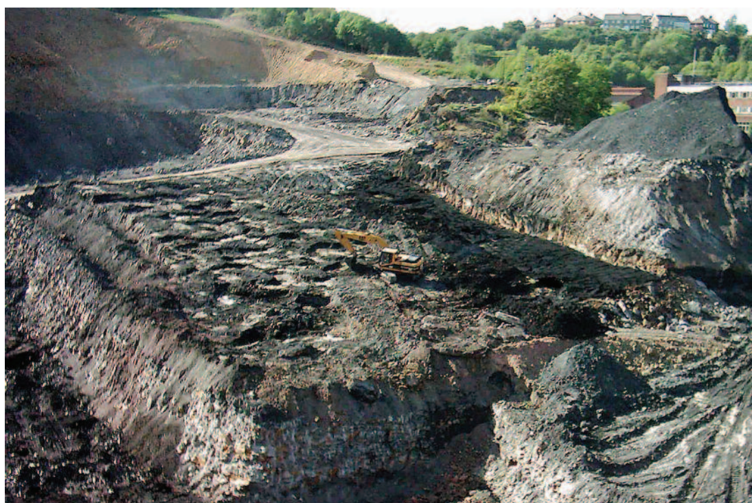
Excavation work during reclamation of the former steelworks at Brymbo revealed coal seams and plant-rich horizons. A mechanical digger (seen centre) is dwarfed by the scale of the excavations. Photo by Jason Parry, Brymbo Developments Limited
