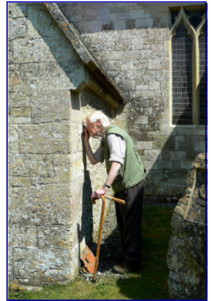
Assessing building stones at Chilmark Church, Wiltshire.
