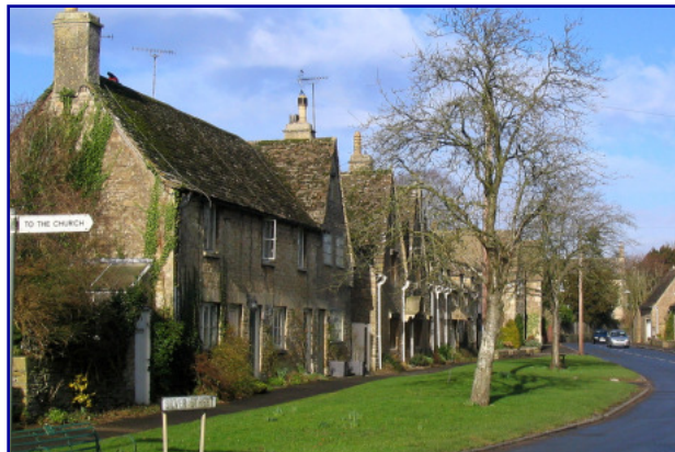
Distinctive Cornbrash is used in many old buildings in the Gloucestershire village of South Cerney.
