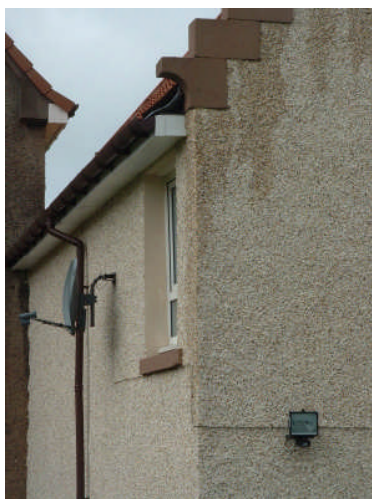
Site in Craigneuk, Airdrie, where - with the agreement of Property Services and the Clerk of Works for North Lanarkshire Council - the triangular fillet on the end of the new pvc fascia was left off to allow Swifts to gain access in 2005. The house in the background shows the usual way of finishing off the verges, with an infill (Photo: © Concern for Swifts (Scotland))
