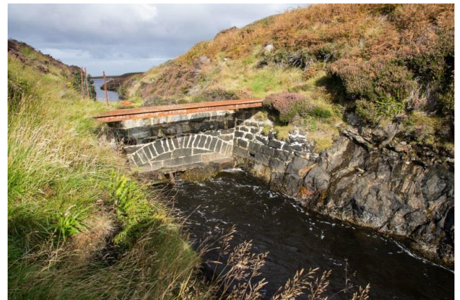
Eastern floodgate and channel from eastern end of Loch Bi.
