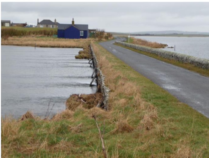
Flap valves on the culverts under the Brig o'Brodgar in Orkney, open to allow flow from the Loch of Harray (right) to Loch of Stenness (left). Photo by Stewart Angus. © +SNH.
