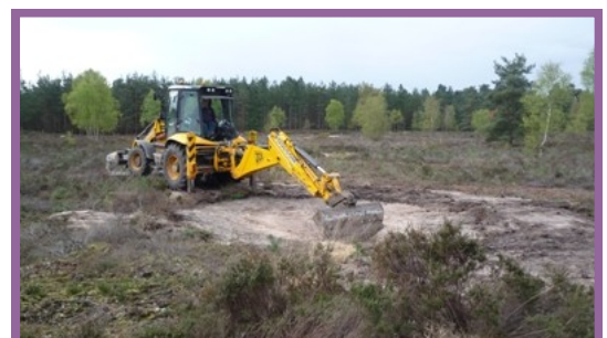
Digging a scrape. Photo: Rob Free (ARC)
