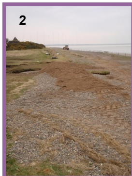
1. Tidal Breach, 2. Filling the gap with shingle, 3. Laying the turves on the top, 4. Staking down the chicken wire. (Above right) The work party. All Photos: Bill Shaw (ARC)
