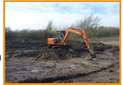
Work in progress with an 8 ton excavator Photo: David Orchard (ARC).
