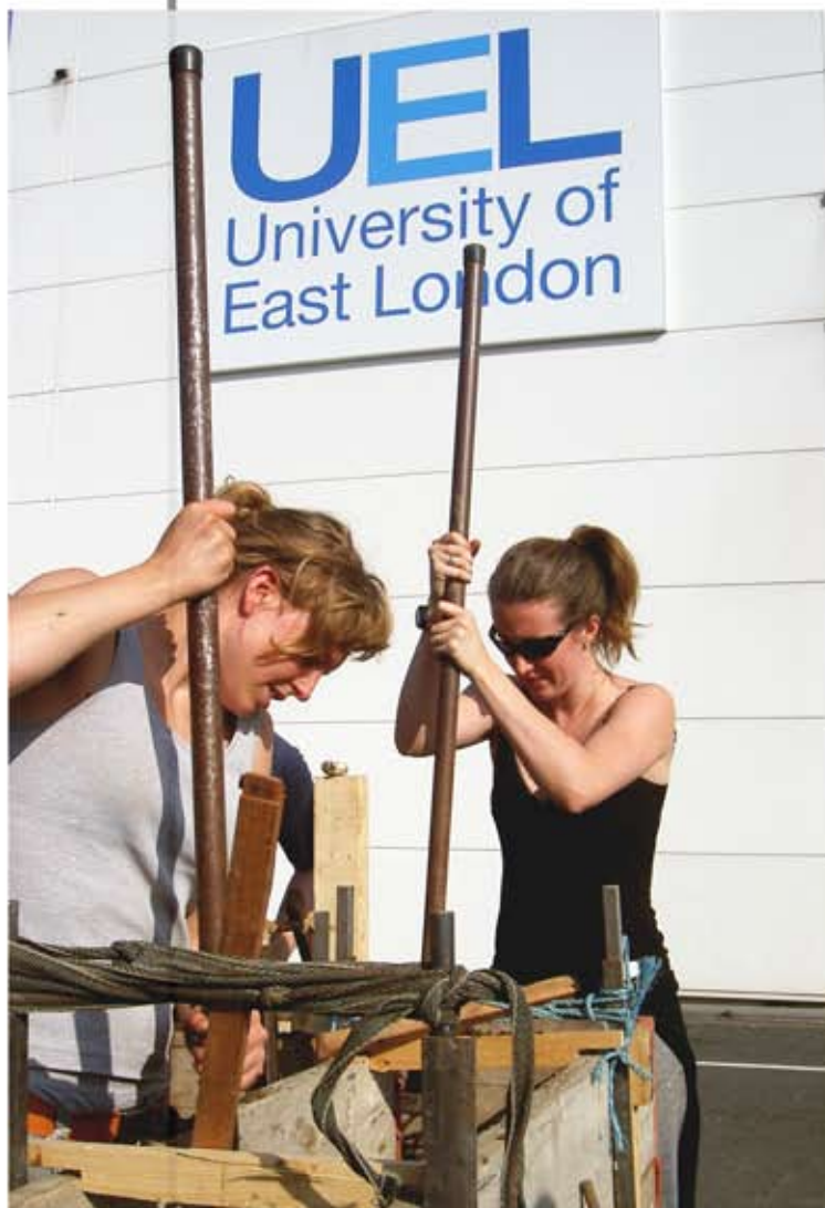
WORKSHOP PARTICIPANTS RAMMING EARTH INTO THE PREPARED FORMWORK
