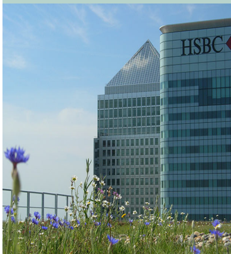
Green Roof of Barclay's Bank, Canary Wharf greenroofconsultancy.com
