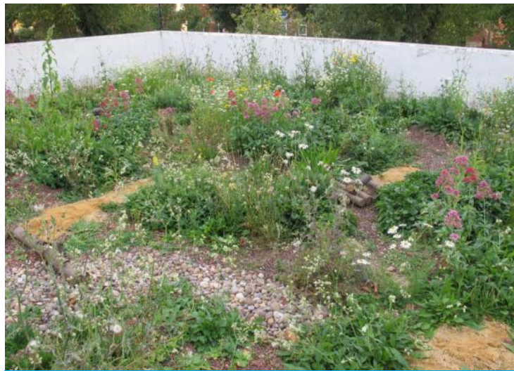
Green Roof on Abbey Hive community building, London © Claire Dinham
