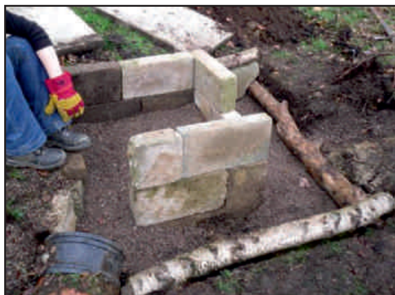
The construction of an artificial otter holt © Emma Rawlings, SWT
