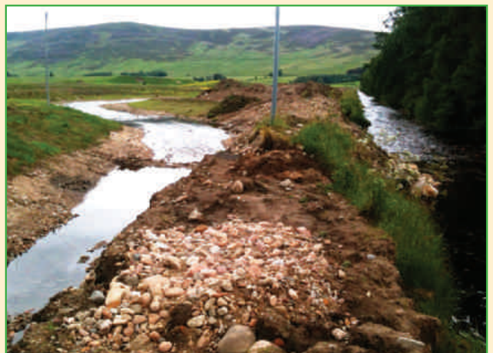
Work on the Rottal Burn, Angus © River South Esk Catchment Partnership
