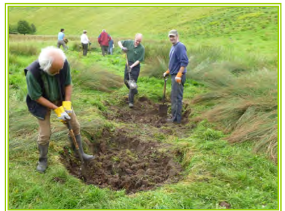
NYCC staff digging one of the ponds. From left to right: Dave Ranner, Matt Millington, Steve Green © Chris McGregor
