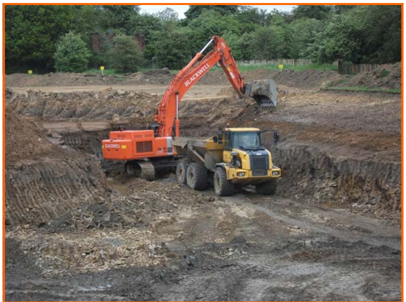
Pond 2 under construction © Wildscapes
