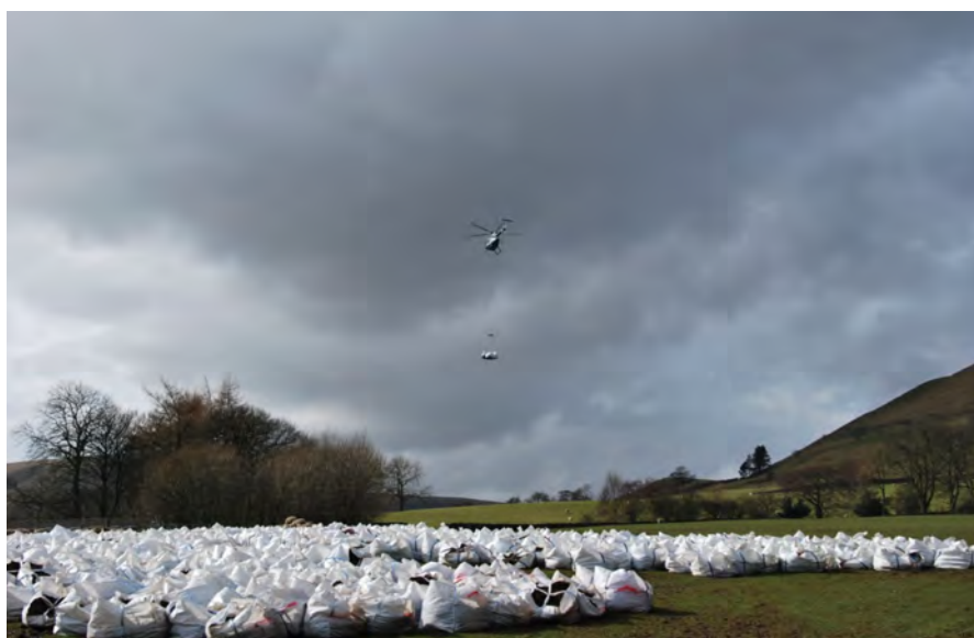
Heather brash bags to be airlifted onto site © Moors for the Future
