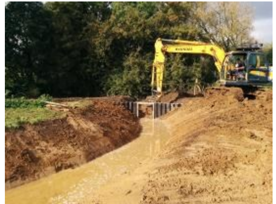
Figure 1: New Control Structure at Little Waltham Meadows © Kieren Alexander
