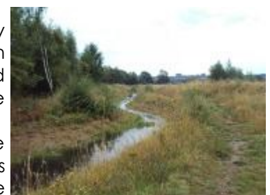
The finished channel - courtesy of Hanson UK
