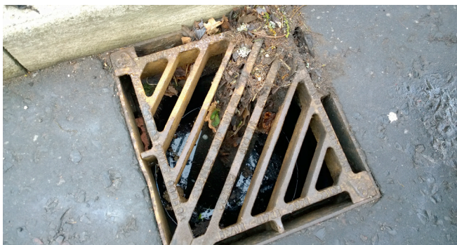
Figure 7. Leaf litter and debris build-up at the ladder top, which facilitates easier escape through the grating. Photo credit: Rose, T.
