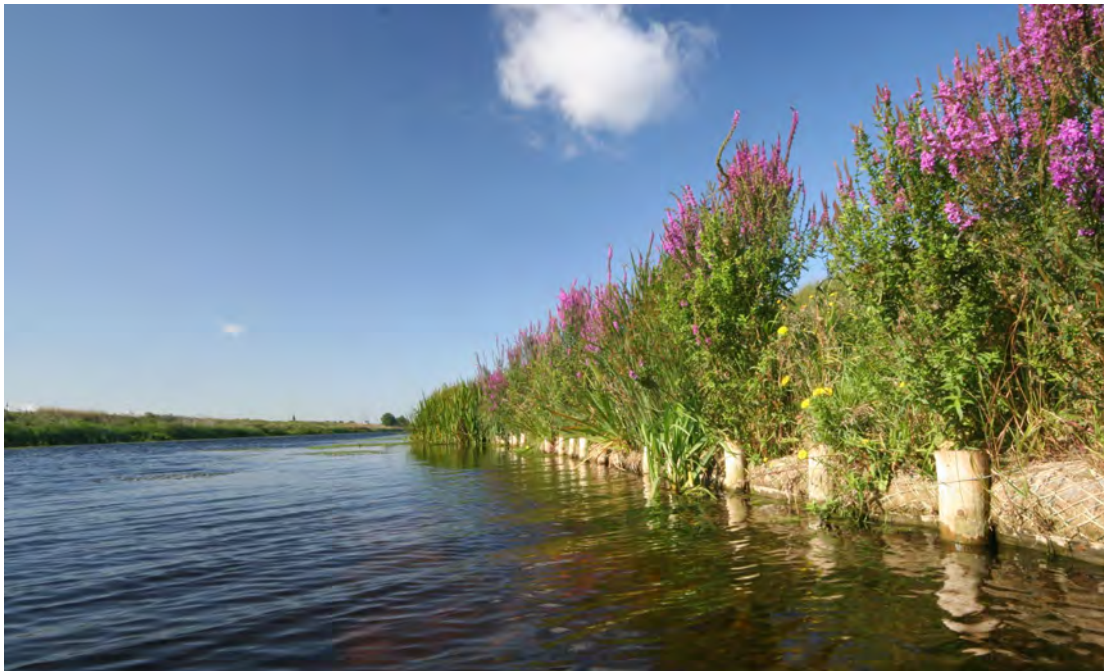
Established coir rolls on the Sixteen Foot Drain near Bedlam Bridge, March East IDB district
