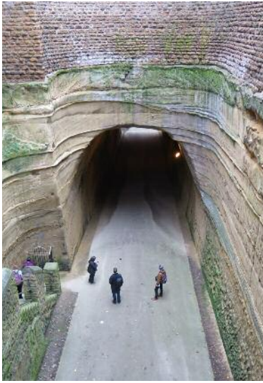
Park Tunnel, Upper College Street, cuts through the Sherwood Sandstone. Photo by Don Cameron
