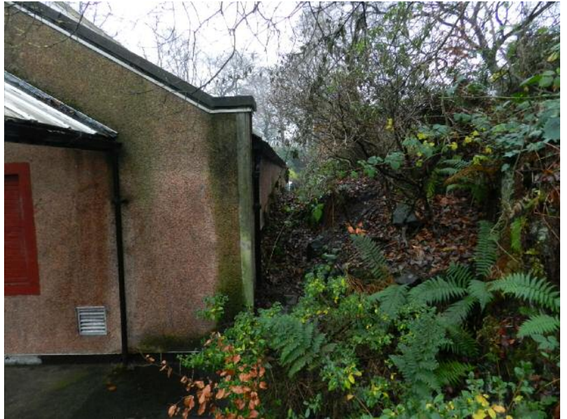
The south side of the Fossil Grove building showing the accumulation of soil and plant debris against the wall. Left to accumulate for years, this material has probably aided ingress of water through the building into the grove.
