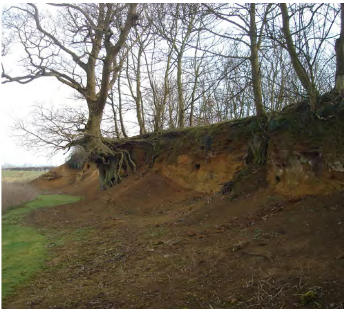
This was the North Face before clearance in February 2011.
