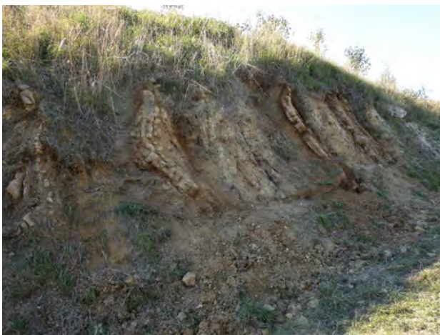
The Upwey cutting during construction in April 2011 (top), in January 2012 (middle) and after conservation work in September 2018 (bottom).
