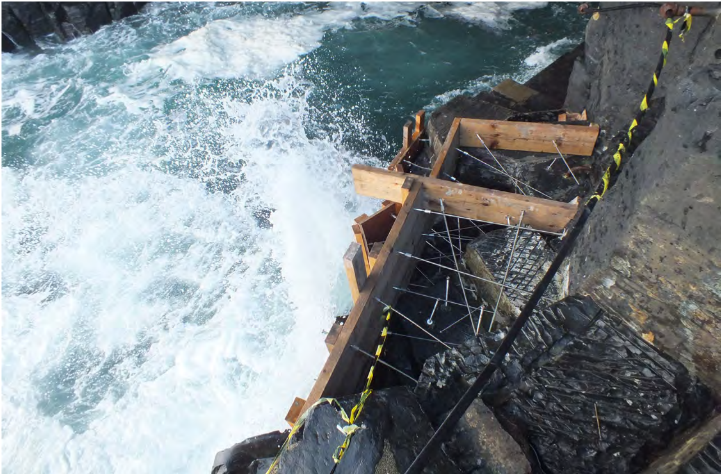
Construction work to restore access at the entrance to Fingal's Cave. Stainless steel rods secure shuttering for concrete, the lower sections of which have been carefully constructed to emulate the geometric forms of the basalt columns. The steel rods also provide a reinforcing element for the concrete © Colin MacDougall
