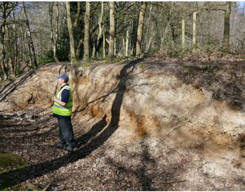
Left: The wall before renovation.
