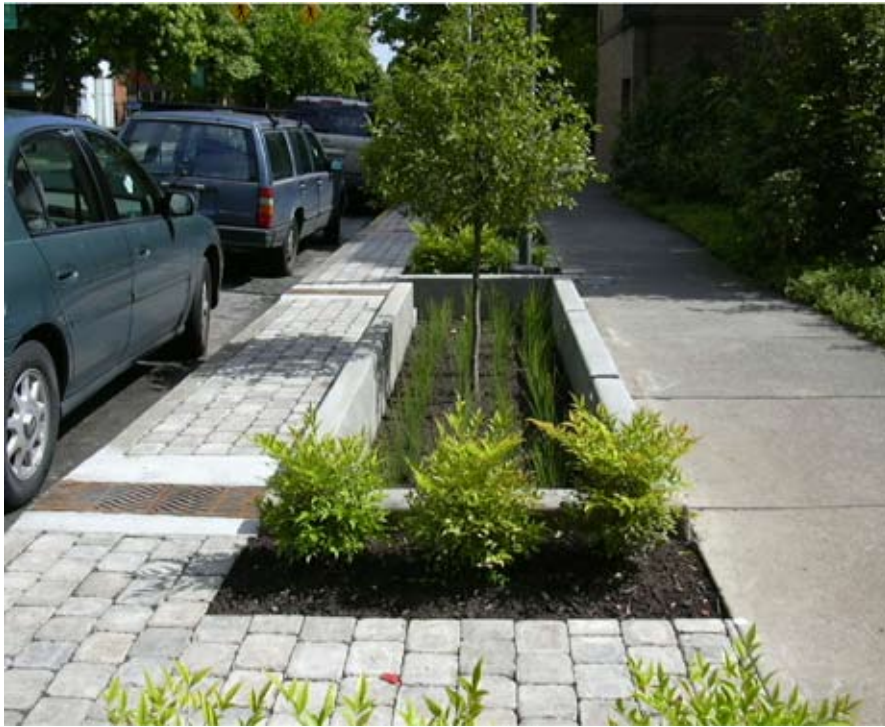
Combined rain garden and tree pit designed to receive run-off from the street.
