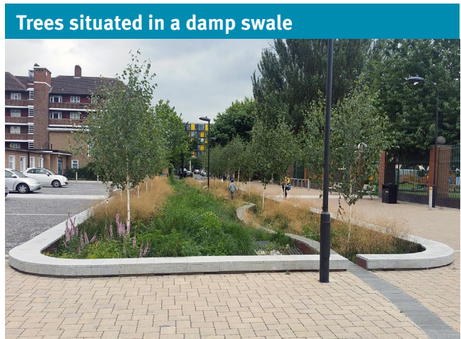
Figure 11. Damp Swale, Joyce Square, London | Robert Baray Associates
