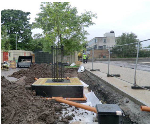
Figure 1. SuDS Dundee Trial Tree Pit | BlueGreen Urban
