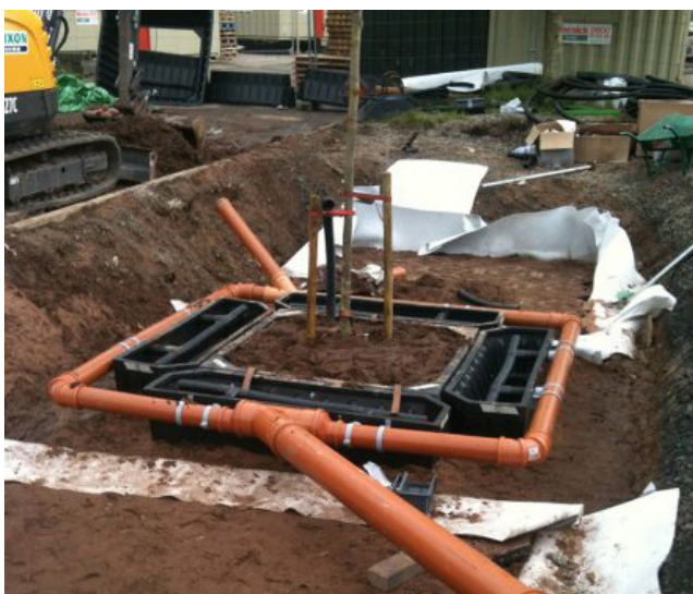
Figure 2. SuDS Dundee Trial Tree Pit | BlueGreen Urban
