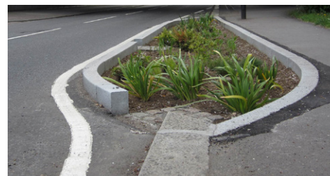
Using a filter strip to reduce pollutants
