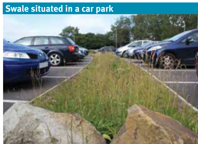
Figure 4. Swale in a car park | CIRIA
