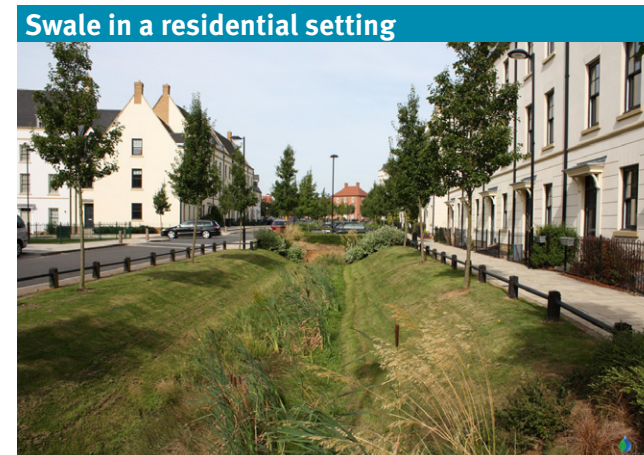
Figure 3. Upton, Northamptonshire | Susdrain, CIRIA
