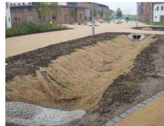
Figure 10. Swale during Construction with erosion prevention | ARUP
