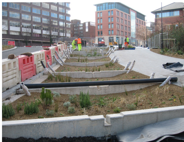
Figure 9. Swale during Construction | Sheffield City Council
