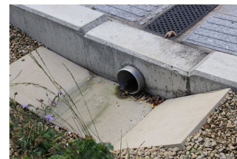
water inlet via a piped connection
