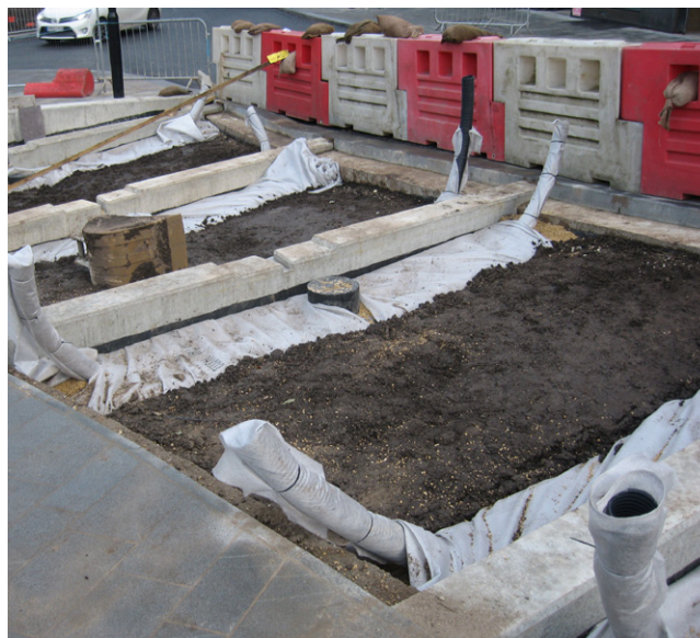
Figure 12. Engineered soil used in rain gardens for Sheffield Grey to Green Scheme | Sheffield City Council
