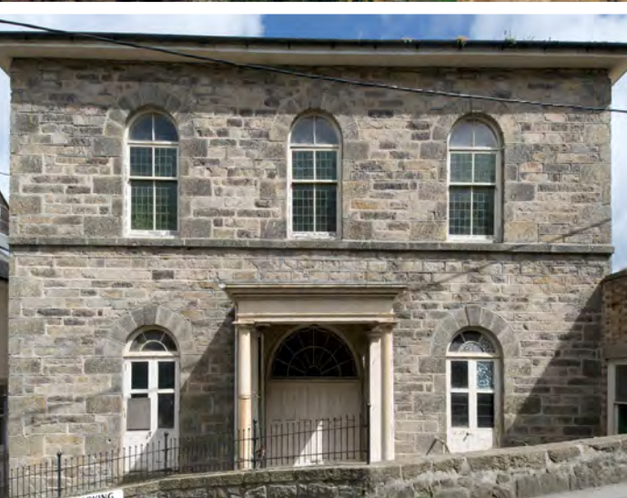
Trinity Methodist Chapel, Newlyn, Cornwall. Building stones: Coursed killas with granite dressings, painted rubble, dry Delabole Slate hipped roof
