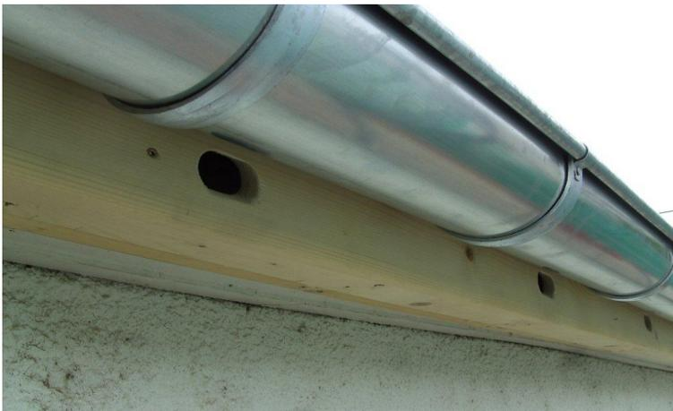
On the left; a simple timber box, with internal partitions, that has been fitted under and behind the gutter to form a continuous array of Swift nest places. The entrance holes are sized to resist access by Starlings.
