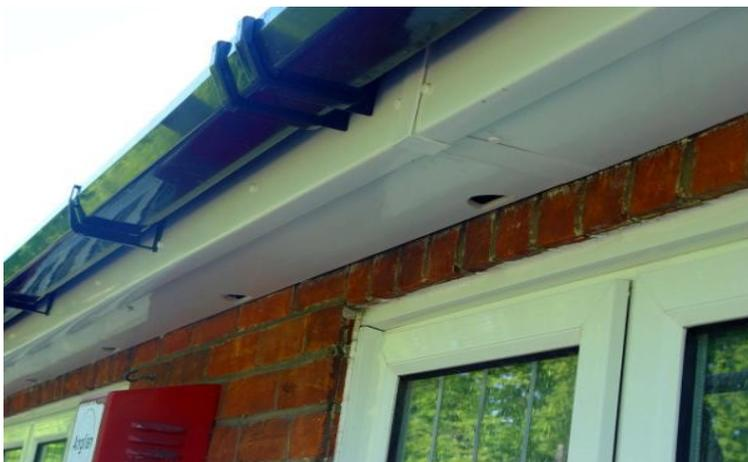
On the left; plastic soffits that have been fitted with internal partitions and drilled with Starling-proof entrance holes for the Swifts to gain access and make their nests inside. These soffits are isolated totally from the roof interior.
