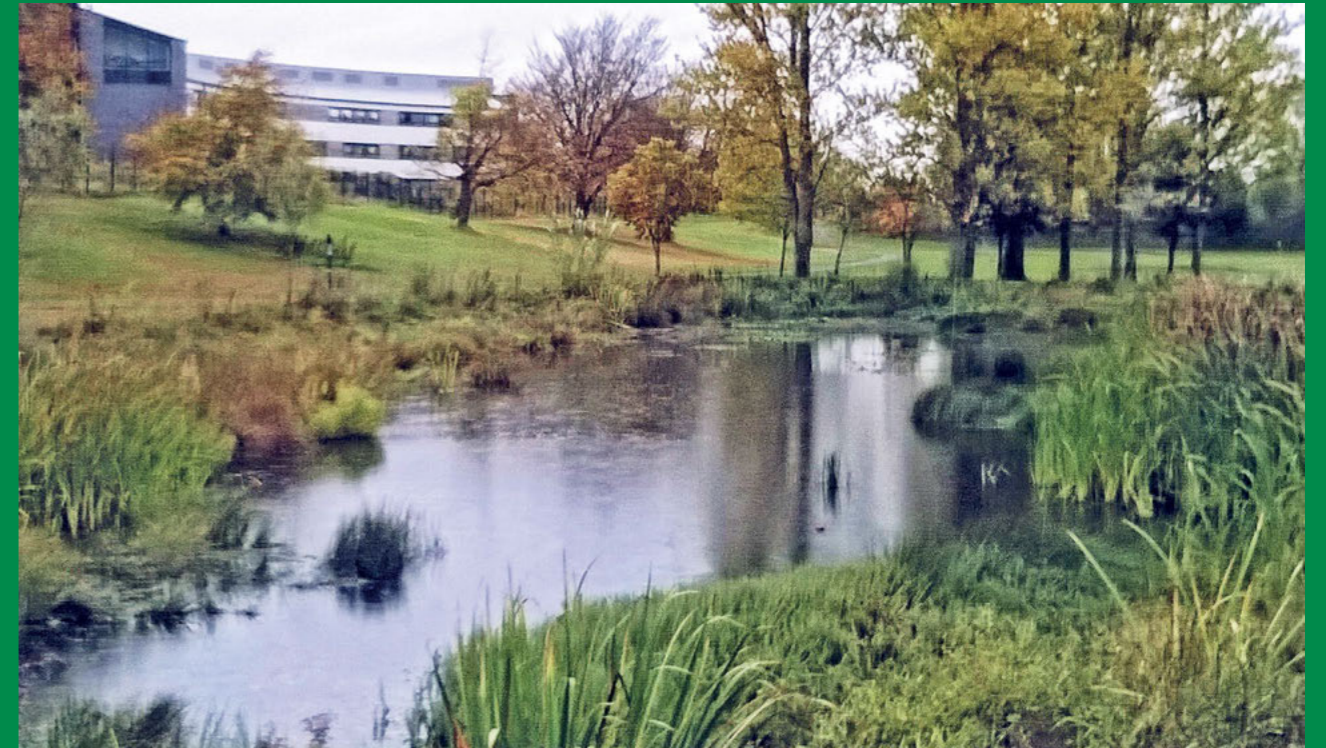
SUDS pond at the North Inch Community Campus in Perth (c) D Williamson
