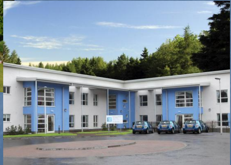
Balhouses Care Home Pitlochry.
