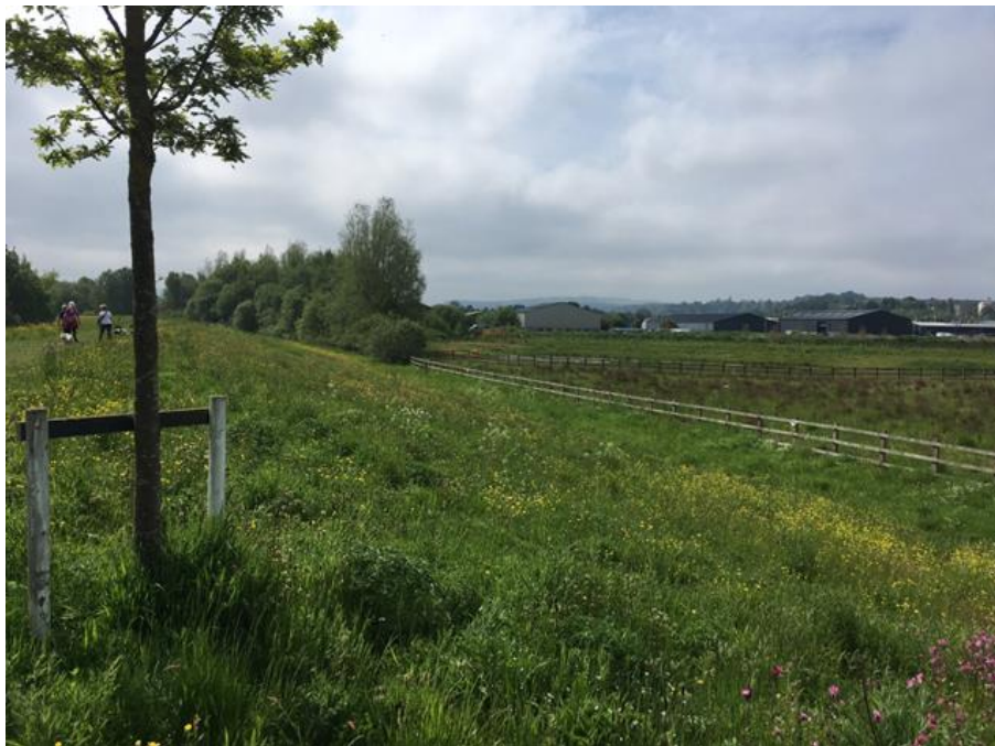
North Muirton Flood Defence grassland, Perth © C A G Lloyd
