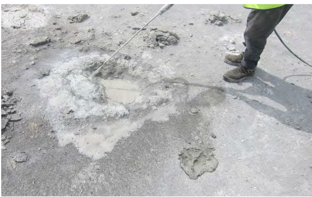
Left: Using a high-pressure lance to clean the surfaces of the footprints.
